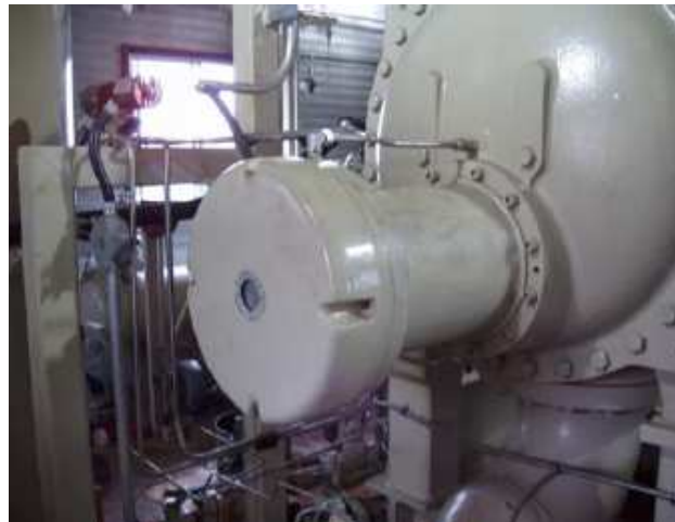
Fig 3: Howden Type Slide Valve
